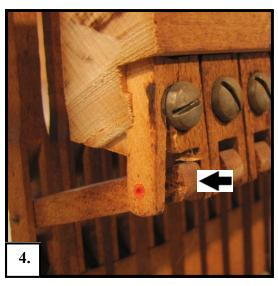
In such a situation, if the action is pushed into place with a bit too much force the lower flange can easily break from the excess pressure, necessitating replacement.
