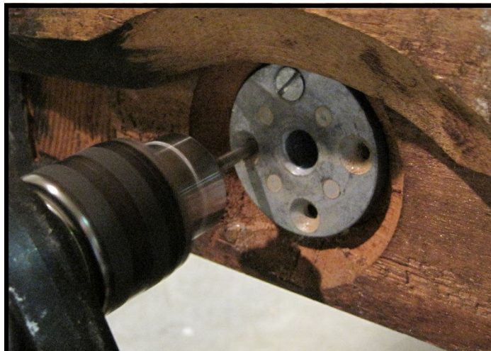
New socket being installed.
